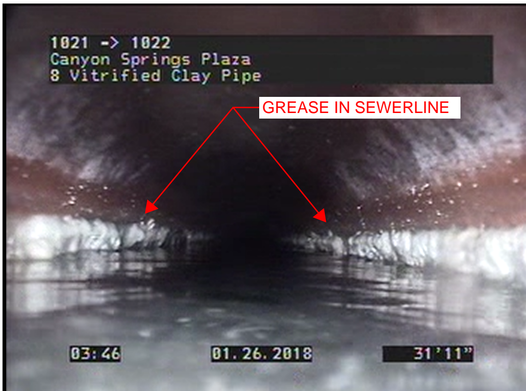
FIGURE 3 - OBSERVED GREASE INSIDE SEWER EDGEMONT COMMUNITY SERVICES DISTRICT CANYON SPRINGS PLAZA
